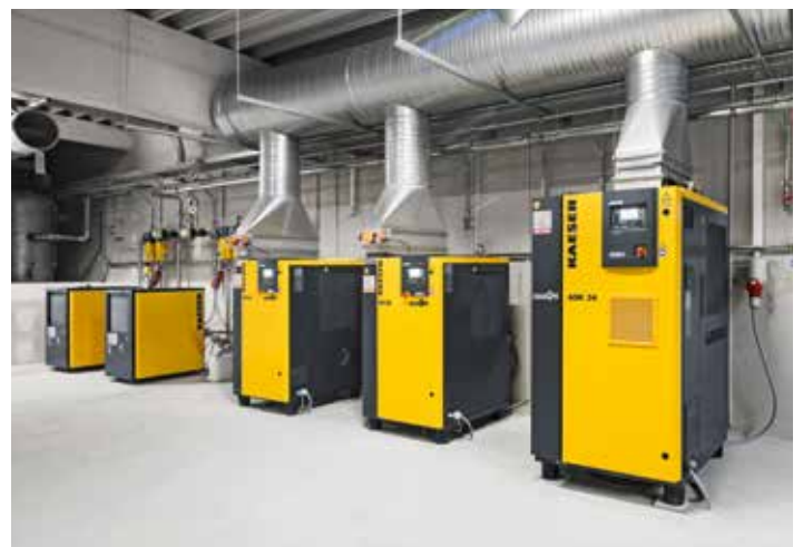
To maintain the required purity class at all times, different sensors transmit their quality parameters to the SIGMA AIR MANAGER 4.0 on a continuous basis.
