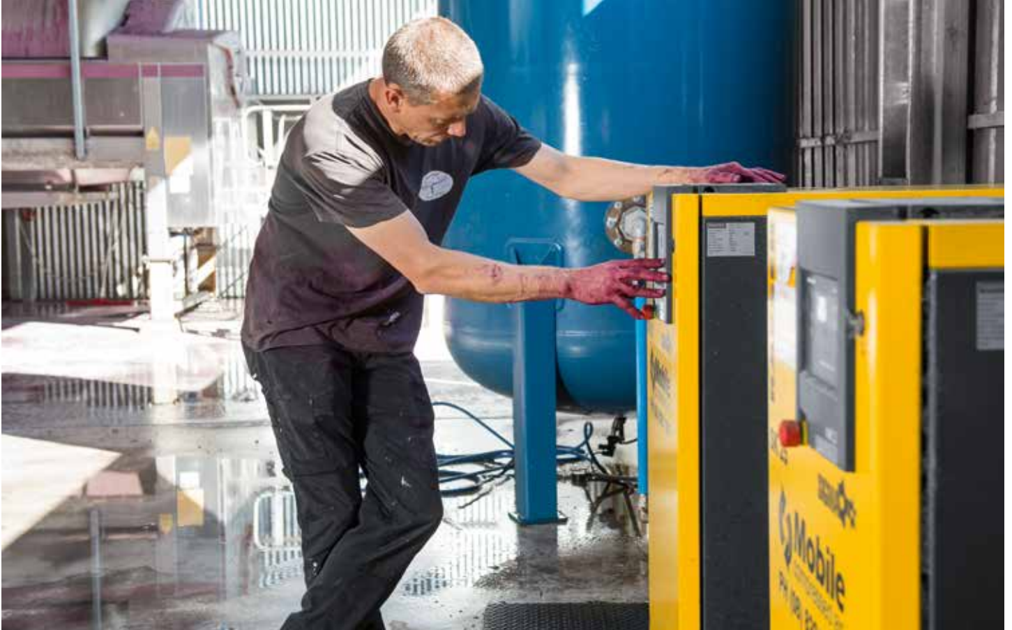
Teusner's new compressed air station: two KAESER SK 25 rotary screw compressors and an air receiver with 5,000 l of storage capacity.
