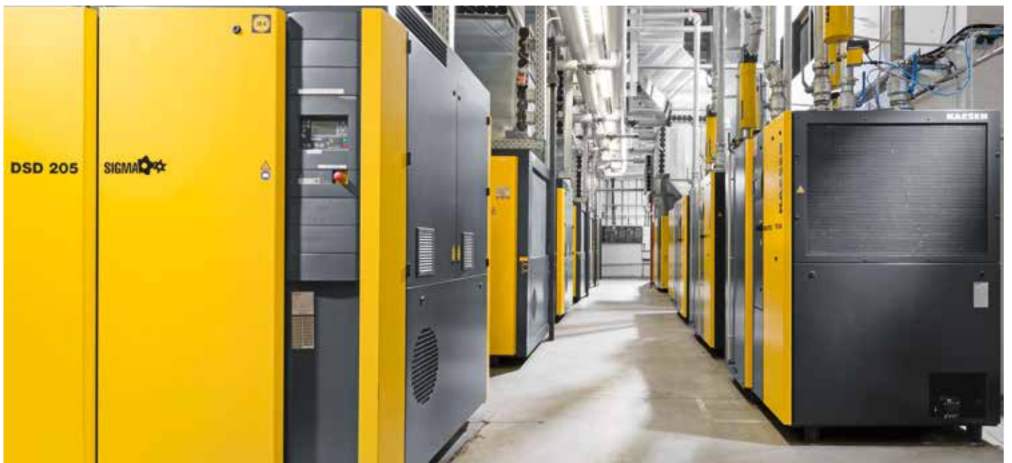
The compressed air production 'Hall of Fame' at nobilia, seen here in plant I.
