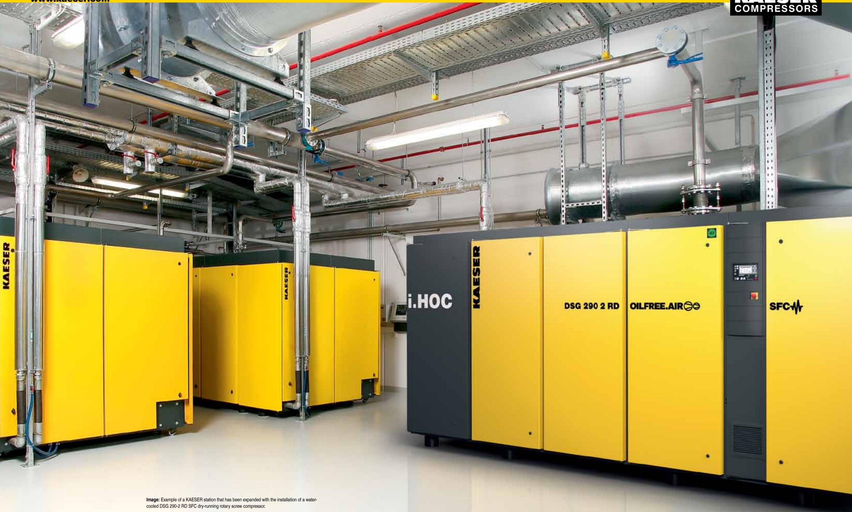
**Image:** Example of a KAESER station that has been expanded with the installation of a water-cooled DSG 290-2 RD SFC dry-running rotary screw compressor.
